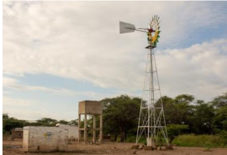
Wells (Windmill pumping)
